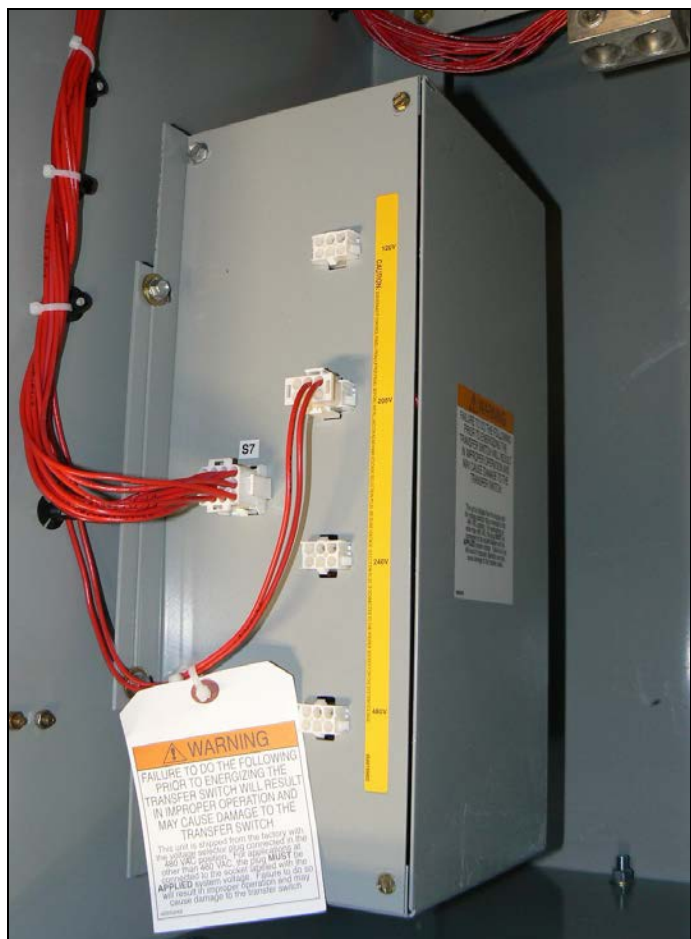
Figure 7. North American Market Voltage Selection Terminals (Shown Connected to the 208 Vac Plug).
